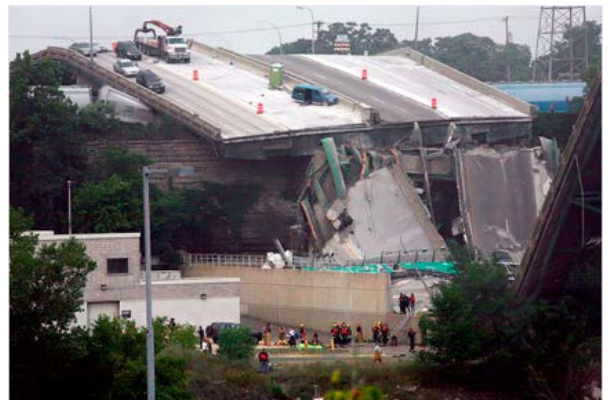
The 2007 Minnesota Bridge Collapse
